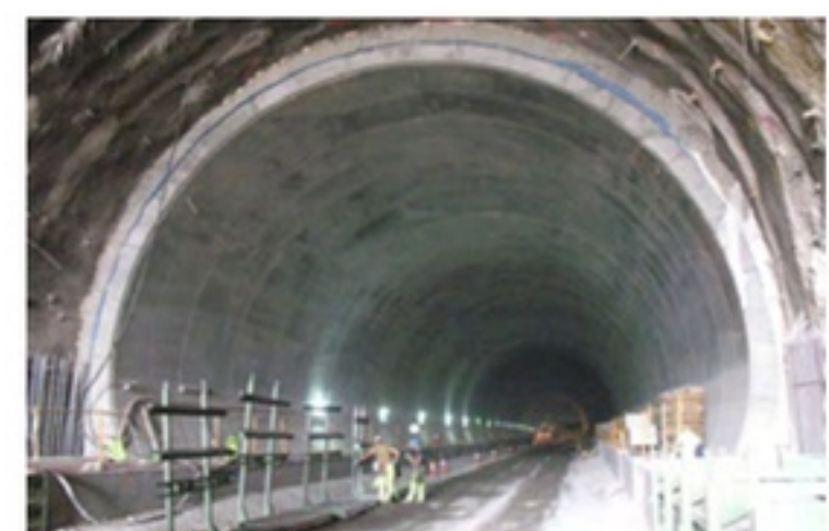
USED IN CAST IN-SITU LININGS
