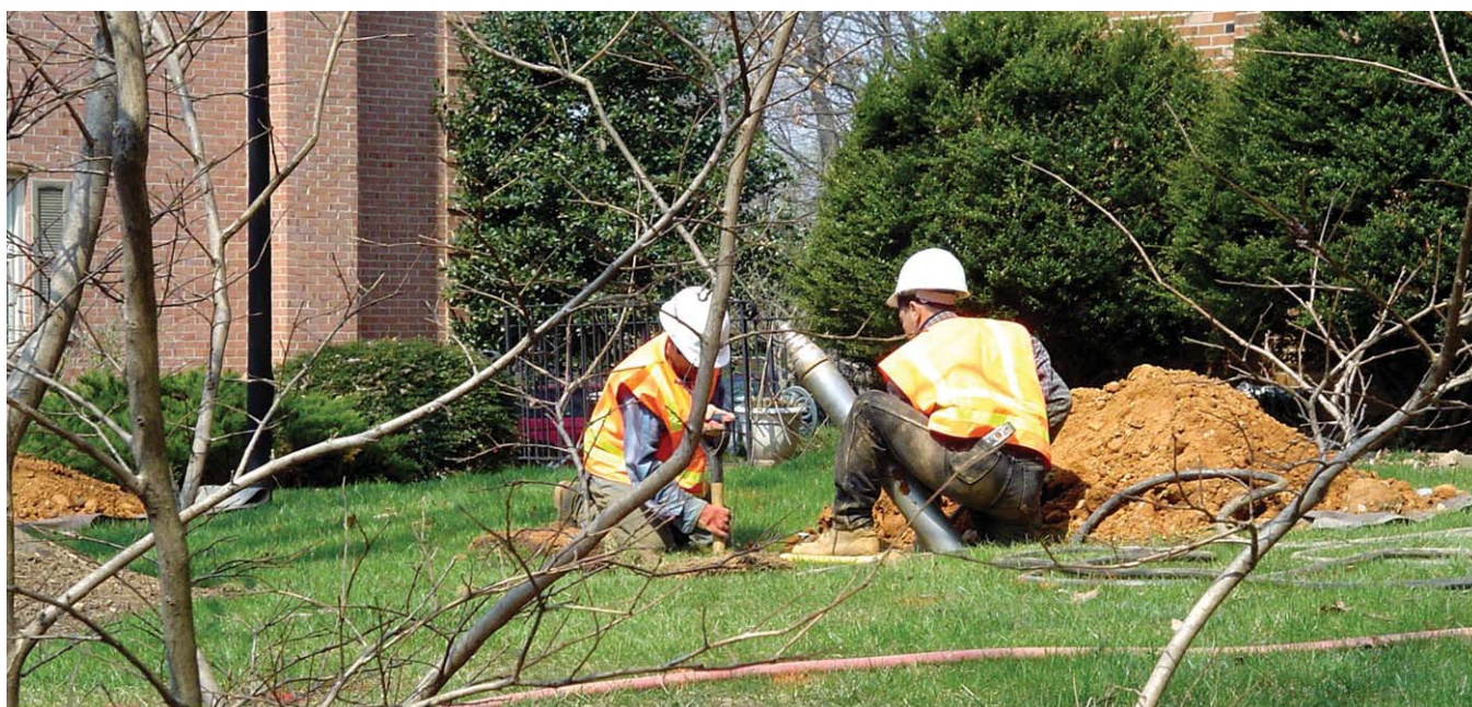
Using an impact mole to install underground cables
