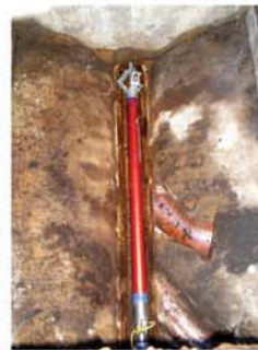
Launching the PipeTrack unit from a manhole.
