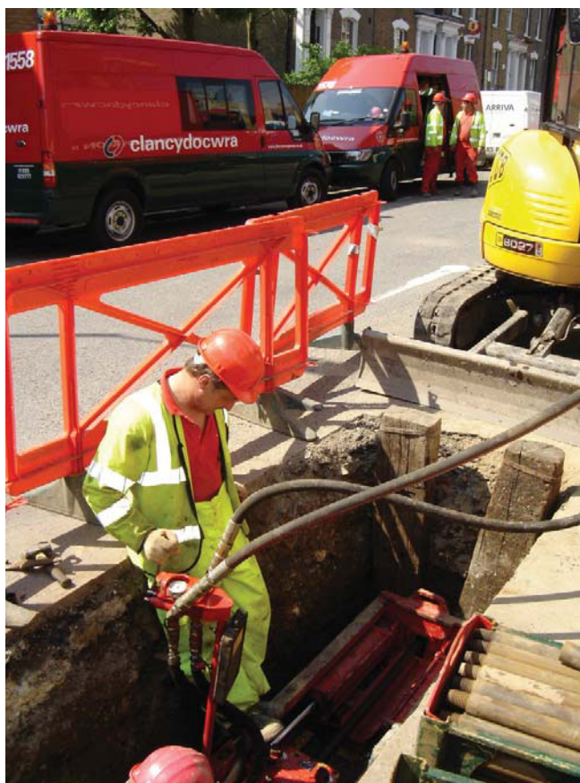
A typical pipe bursting rig in operation
