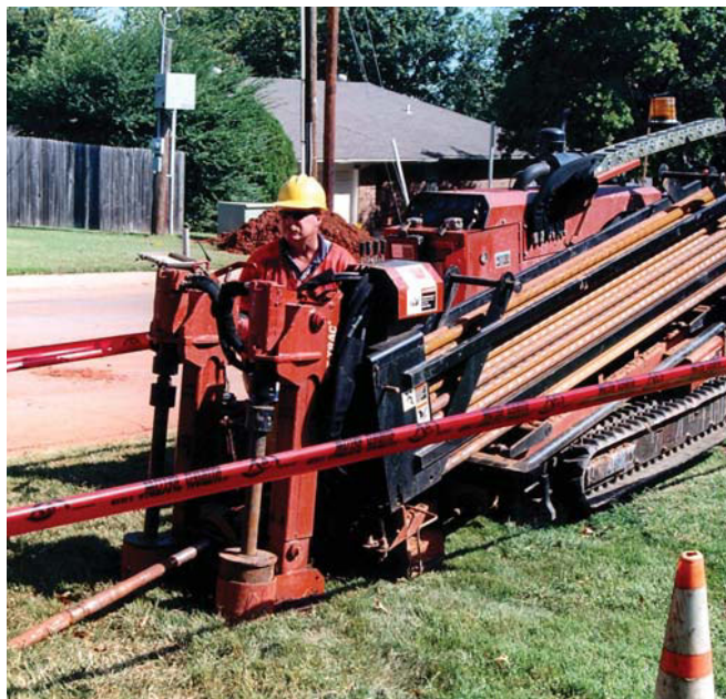
HDD drilling rigs being used to install cables or cable ducting underground in the USA
