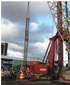
Installation of reinforcement on the East Shaft
