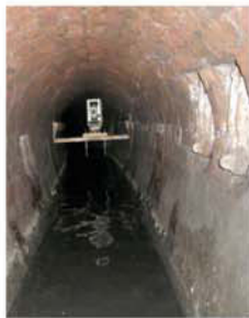
A total survey station in a main sewer.
