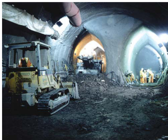
Heathrow Express crossover, which was constructed using sprayed concrete
