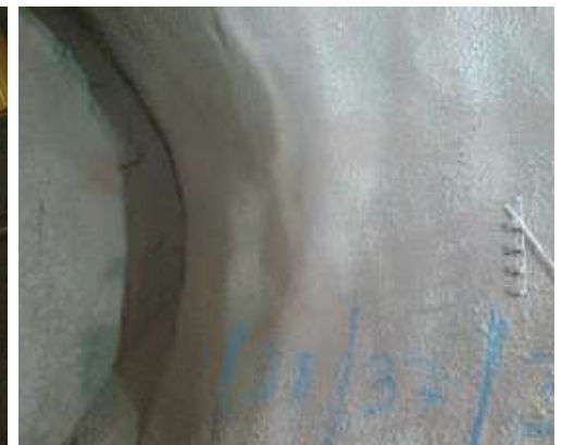
Figure 4: A normal digital photograph of a shotcrete lined tunnel
