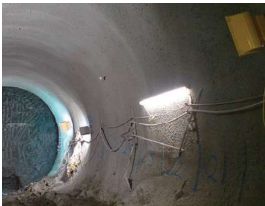
Figure 2: View of a tunnel lined with shotcrete
