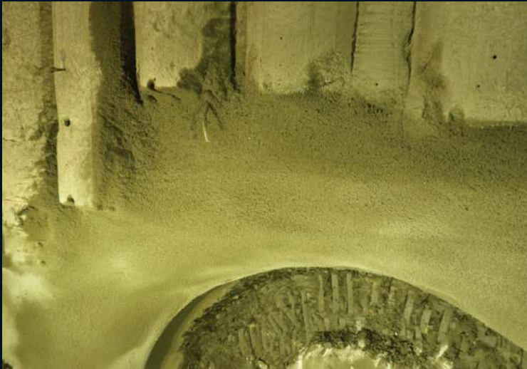
Figure 6: Digital image of enlargement top heading advance 1
