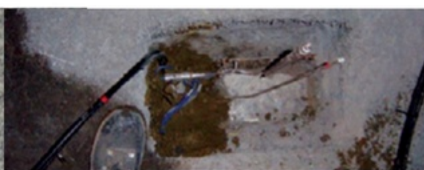
Figure 3 (left): One of several multicore cables required for 2 arrays of instrumentation (pressure cells and strain gauges) installed at Heathrow Terminal 4 station in 1996 (photo taken in 2015)
