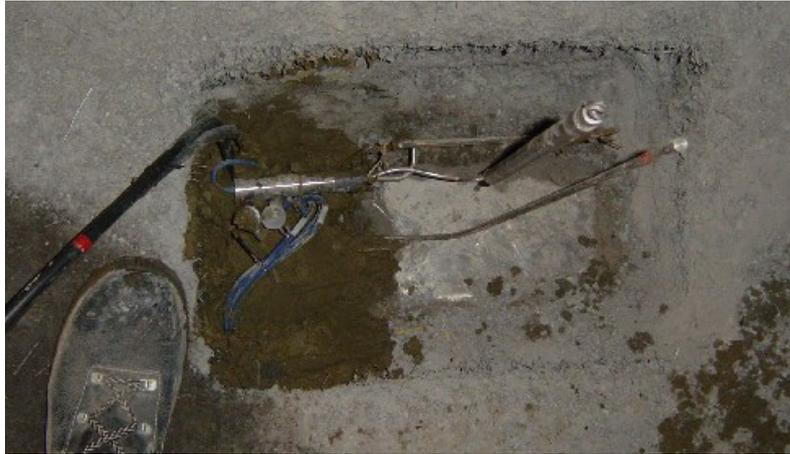
Fig. 3: Installation of radial and tangential pressure cells within a box-out of the sealing layer.
